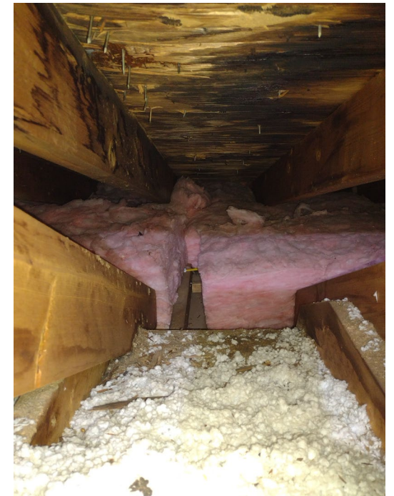
Roof leaks
