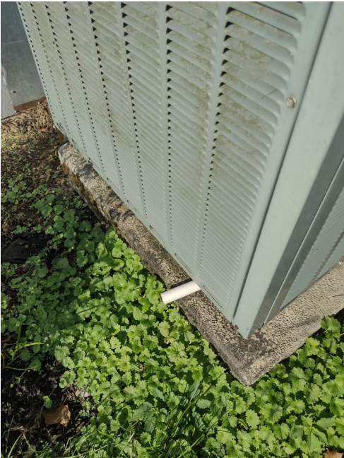
Condensate line / pump
