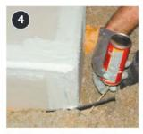
Seal box on all sides and edges to make continuous barrier from attic.
