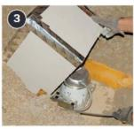
Premade boxes can make installation easier when installation site is clear of framing members.
