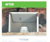
When boxed with appropriate clearances and fire-rated materials, fire risk is mitigated and air leakage is reduced.
