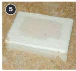
Top of box must be R-1 or less and left free of insulation. Flag enclosure for added visibility.
