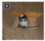
Clear any debris and insulation from around non-IC rated can light.
