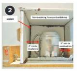
Enclosure has 3 inches of clearance from lamp to insulation on all sides.
