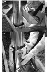
Sealing manufactured chimneys: When installing retrofit insulation in addition to air sealing, install a shield on top of the air seal that extends above the level of the new insulation.
