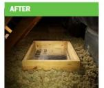
Safely and durably sealing and insulating attic access doors prevents air movement and reduces heating and cooling loads.
