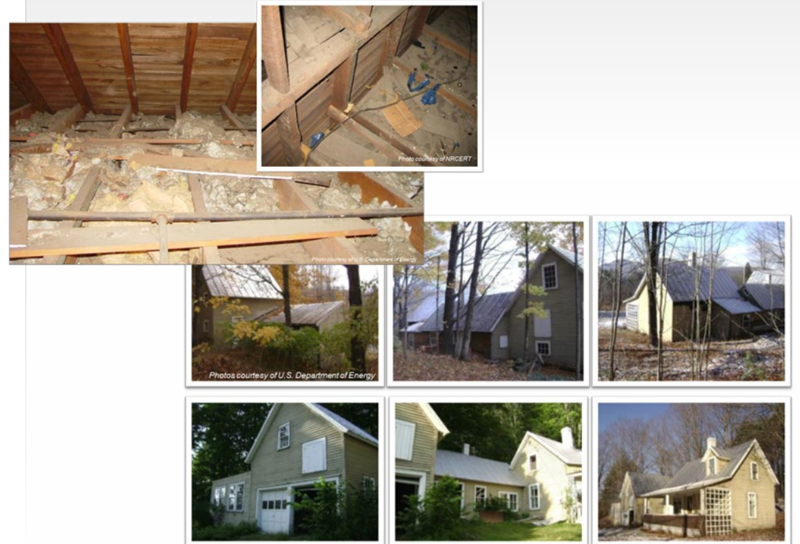
Figure 13: Example detail photos documenting existing conditions
