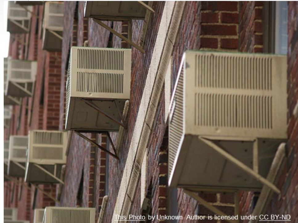
Figure 12: Window/room air conditioners installed in residential building
