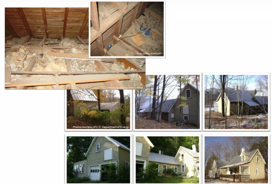
Figure 13: Example detail photos documenting existing conditions
