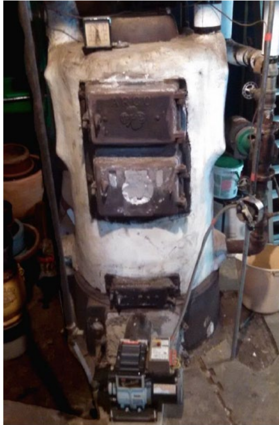
Boiler wrapped in asbestos insulation Picture from Expanded HEAT Loan Initiative Report , December 2015, E4TheFuture.
