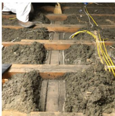
Remove existing 1. insulation
