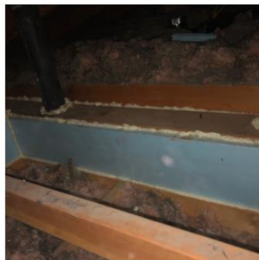
6. Air seal chases, drop soffits
