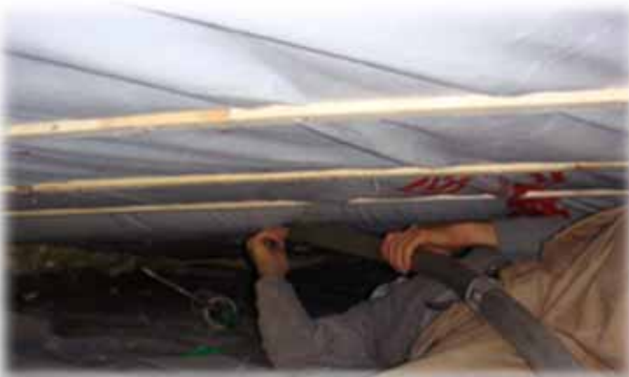
A weatherization technician installs blown in insulation into the floor system pictured above.
