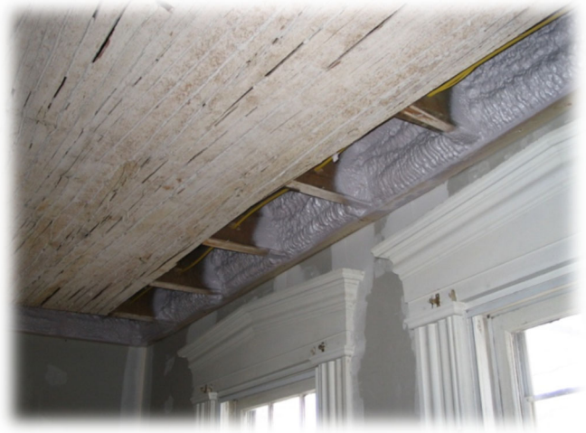
Above, self-help project components enabled the rim (a 6" beam) to be included in the Wx project.
