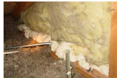
Figure 2122-3: Stud cavity sealed with 2-part spray foam
