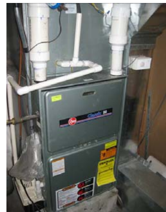
Figure 3133-1: Direct vent sealed combustion furnace
