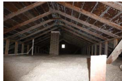
Figure 2122-8: Cut-off chimney in attic
