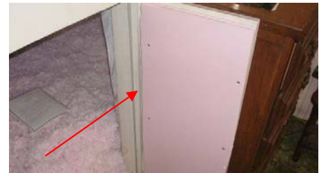
Figure 21365-1: Knee wall hatch insulated and weatherstripped
