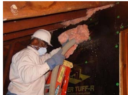
Figure 21364-3: Knee walls being dense-packed with cellulose
