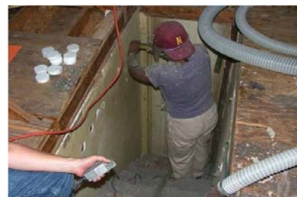
Figure 2135-3: Stairwell walls being dense-packed
