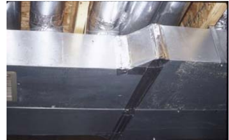
Figure 3124-1: Repair duct system
