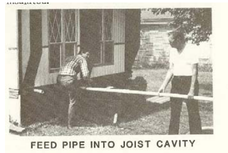
Figure 41421-2: Blowing a mobile home floor from the front
