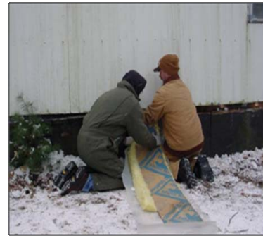
Figure 41521-1: Batt-stuffing a mobile home wall
