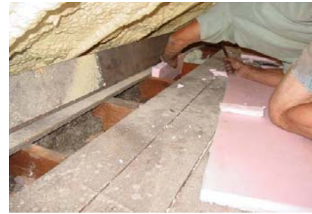
Figure 21364-4: Connecting roof thermal boundary to sidewall thermal boundary with rigid foam board insulation; 2-part spray foam will also work
