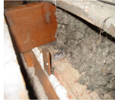
Figure 2122-6: Fur cavity sealed with 2-part spray foam
