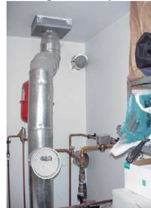
Figure 3124-2: Combustion air intake
