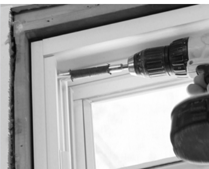
Block frame window installation: Block-frame windows don't have a fin. Installers use plates or screws to fasten the window to its opening.
