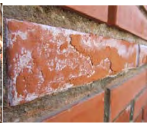
EFFLORESCENCE & SPALLING
