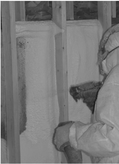
Spraying open-cell foam: The sprayed open-cell foam is left short of filling the cavity or else shaved off.
