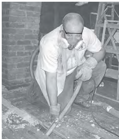
Finished attic floor: Find the large air leaks underneath the flooring and seal them before insulating the space between the joists.
