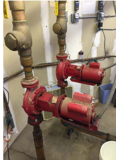
Figure 40 – Space Heating Circulation Pumps
