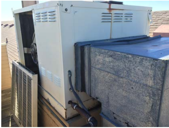
Figure 43 – Evaporative Cooling w/ Unit Heater
