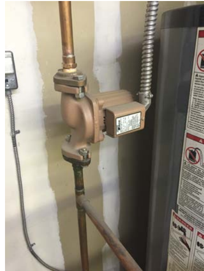
Figure 42 – DHW Circulation Pump
