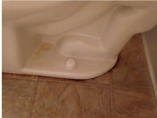
Figure 46 – Potential mold around base of toilet
