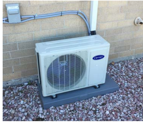
Figure 44 – Ductless Split (Outdoor)
