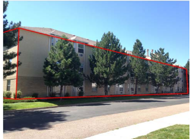
Figure 14 – North & East Thermal Boundaries
