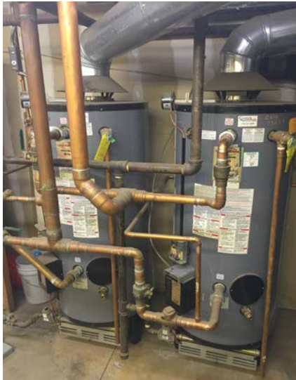
Figure 41 – Domestic Hot Water Heaters
