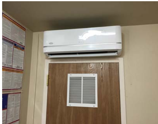
Figure 45 – Ductless Split (Indoor)
