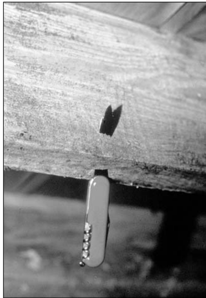
Rotting wood is fragile and dangerous, as this pocket knife test shows.
