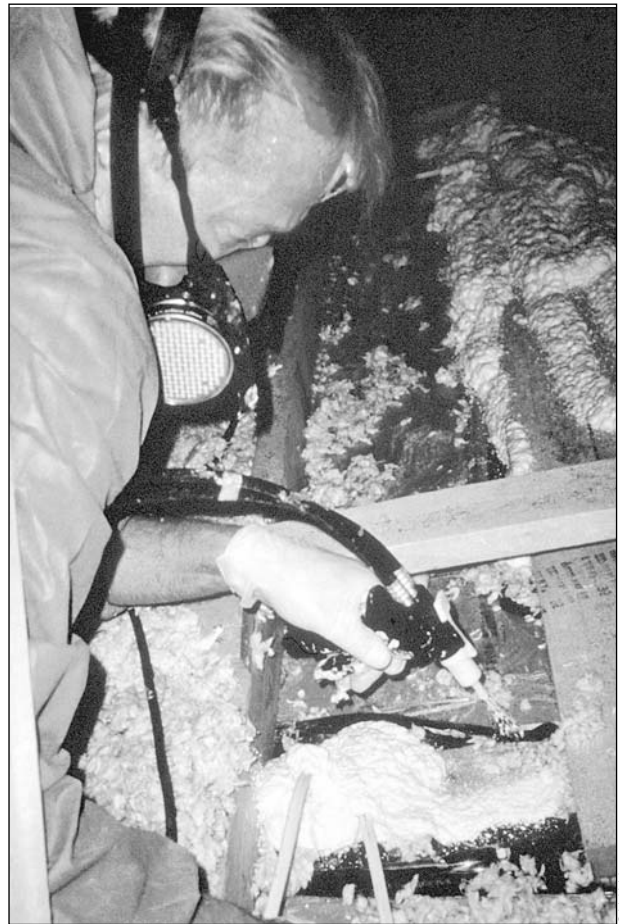
The crew lays continuous beads of foam to seal all leaks.
