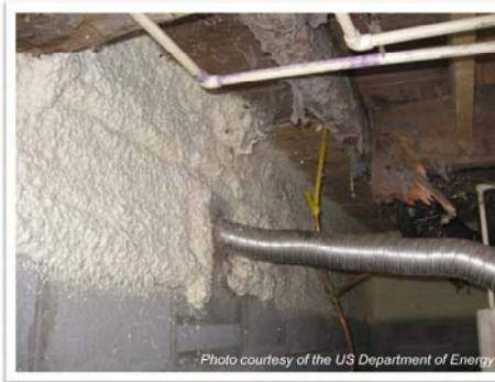
Two part foam insulation on basement wall.
