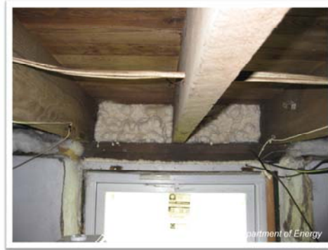
Perimeter air sealing and insulation with two part foam.
