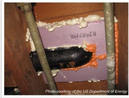
Sealed plumbing penetration.
