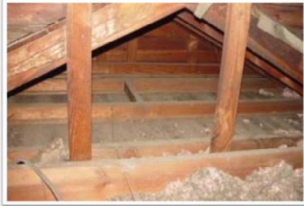
An uninsulated attic ...
