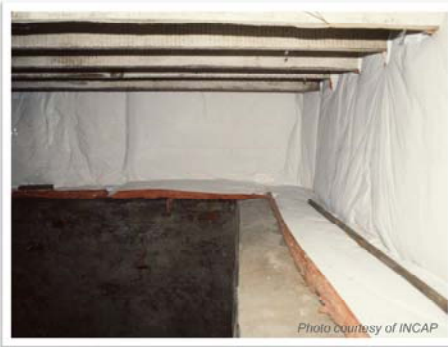
Insulation on crawlspace foundation.
