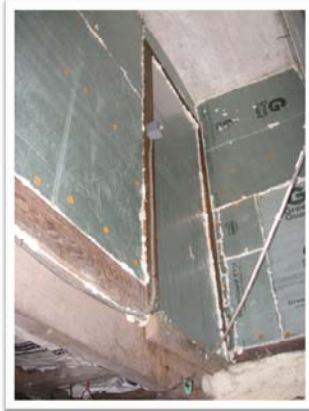
Great air sealing job on old basement stairwell.
