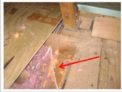
Properly sealed partition wall prior to insulation.
