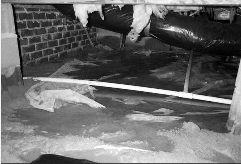
An unusual amount of rain, as well as thin brick veneer walls, resulted in this crawlspace being flooded.
