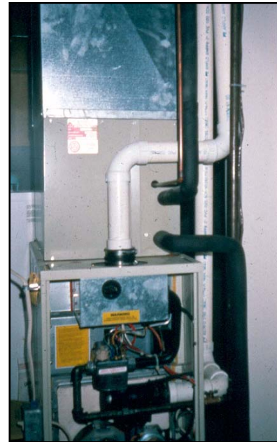
This direct-vent, sealed combustion gas furnace does not require worst-case draft testing
