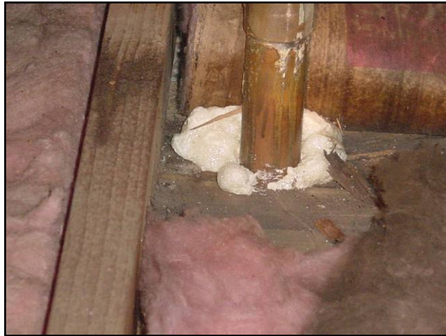
Plumbing stack sealed with foam
