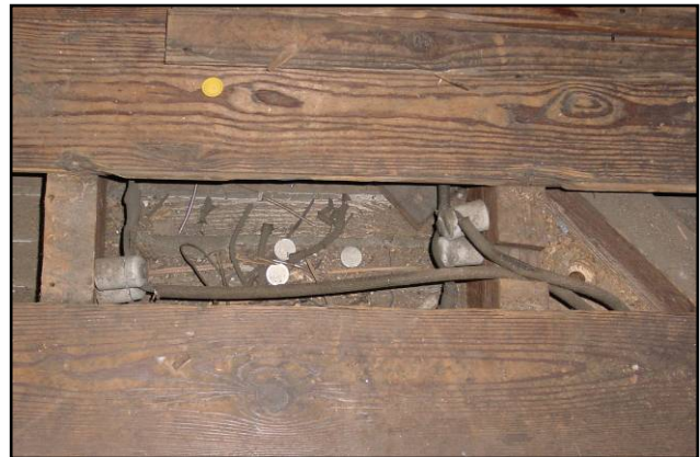
Knob-and-tube wiring can be hidden under attic floors; don't forget to inspect for it and then treat it accordingly
