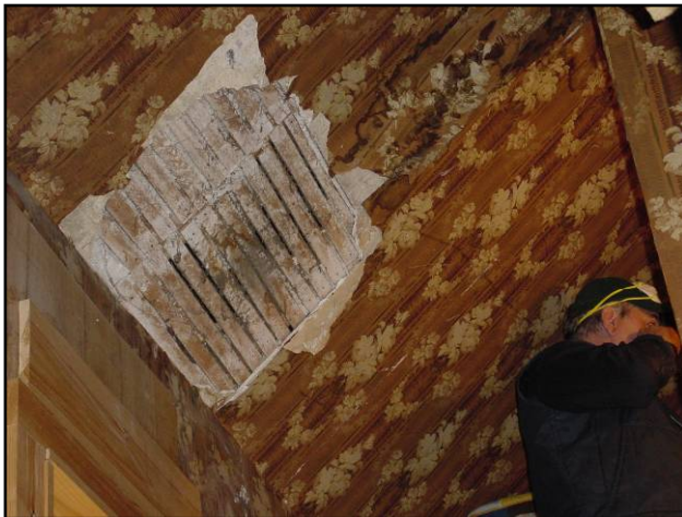
A significant air bypass in a closet up into a sloped ceiling through plaster and lath
