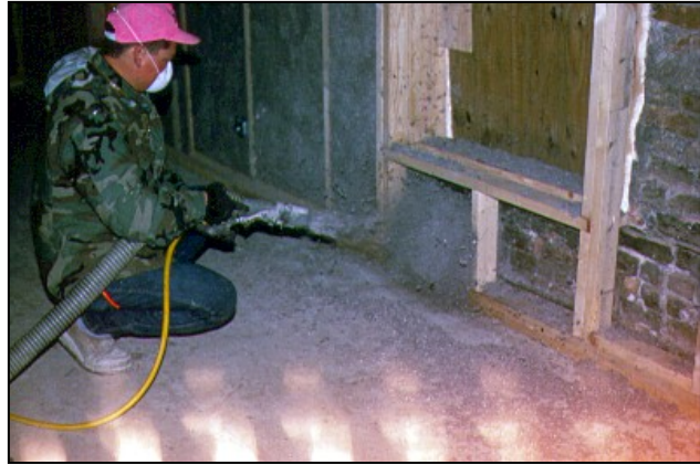
Wet spray cellulose being installed
