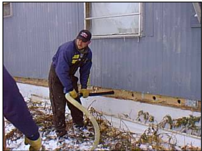
Blowing a mobile home floor
