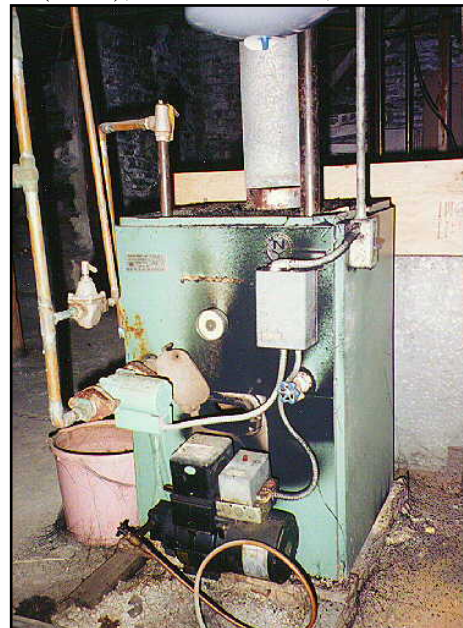
Obvious evidence of drafting failure
