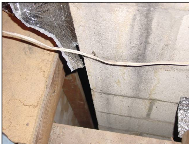
Foil faced bubble wrap may NOT be used for sealing chimney chases.
