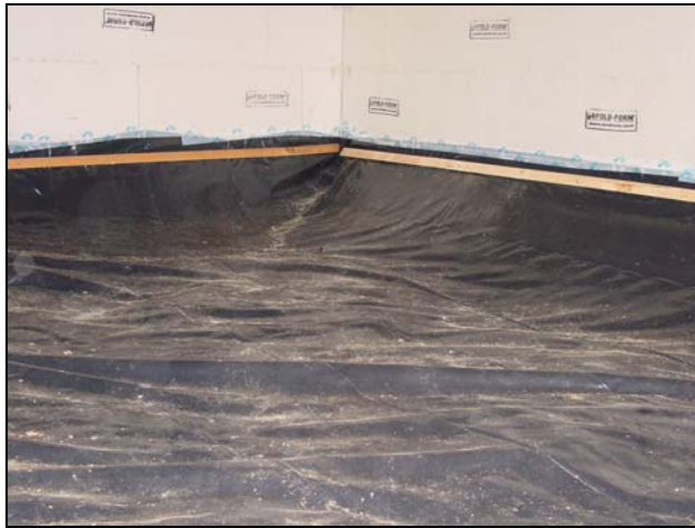
Ground cover sealed to foundation walls
