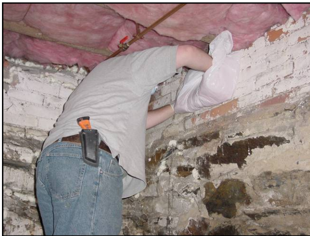
Stuffing the band joist area with an “insulation pillow” (a plastic bag filled with fiberglass)
