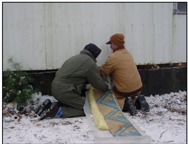
Batt-stuffing a mobile home wall cavity
