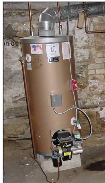
Oil-fired water heaters are not common
