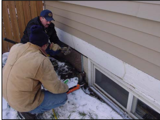
Installation of rigid exterior foundation insulation
