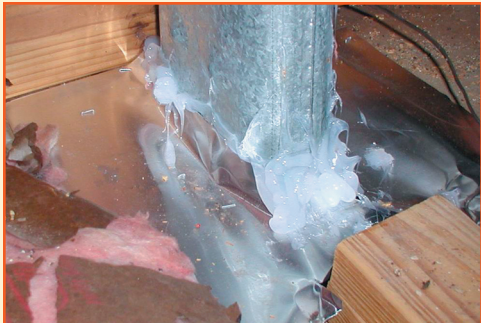
Use two-part urethane foam to air seal cracks and joints. Use high-temperature caulks (clear type is shown but red type is more widely available) around chimneys, vents, and other hot surfaces.
