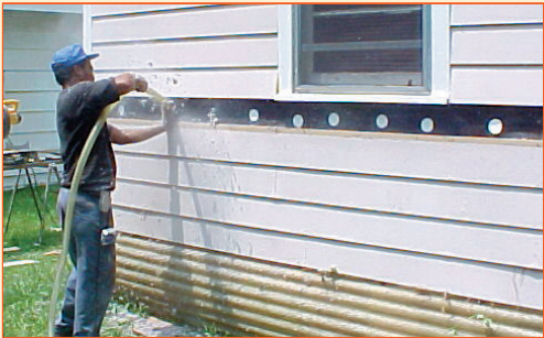
Push the tube into each cavity. Slowly pull the tube out as the flow of insulation slows.
