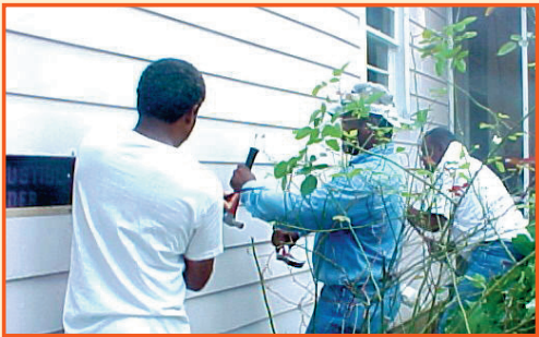
Remove siding and drill through sheathing to access wall cavities.
