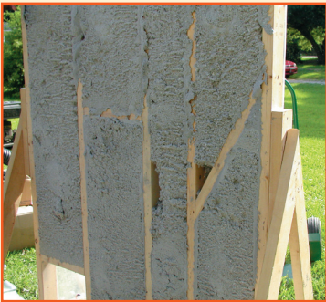
Practice installing dense-pack sidewall insulation on a wall mock-up to learn the tricks for completely filling cavities.
