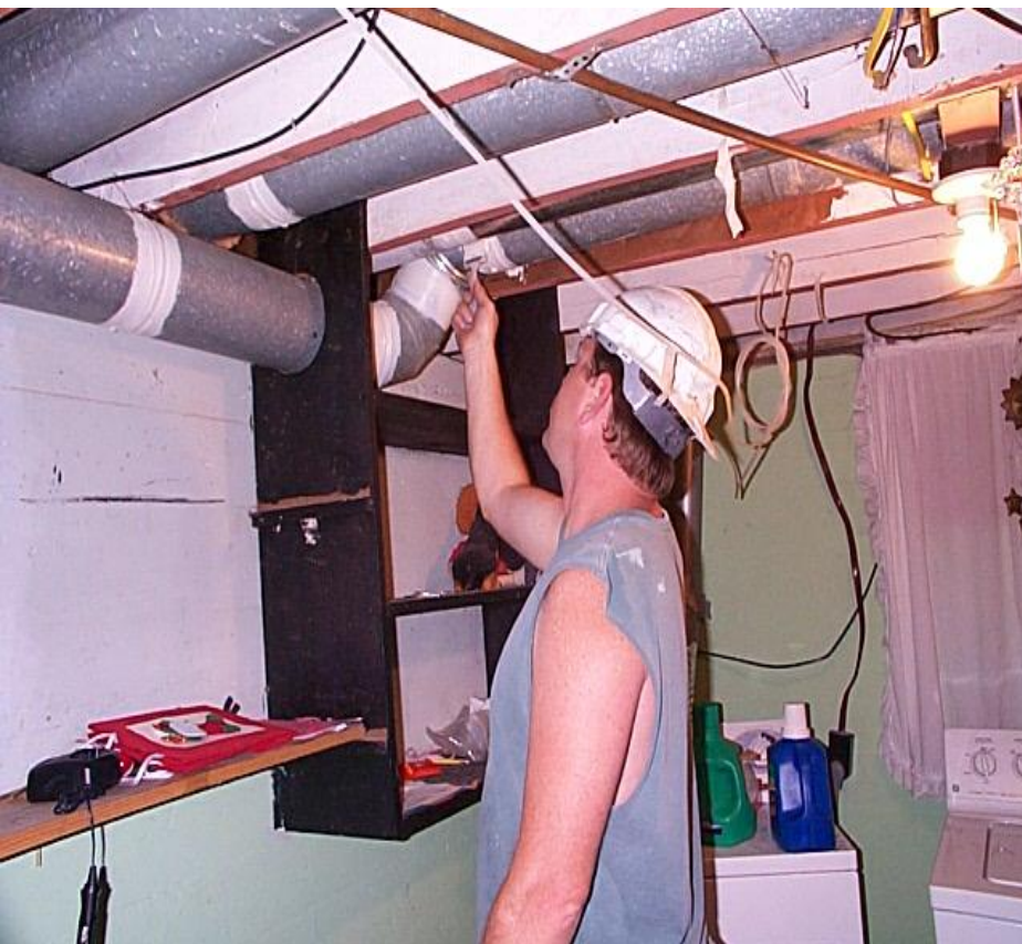
Seal leaking Joints
