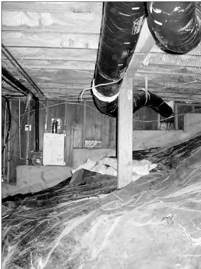
A poly barrier is being put in place to reduce moisture migrating from the soil surface.
