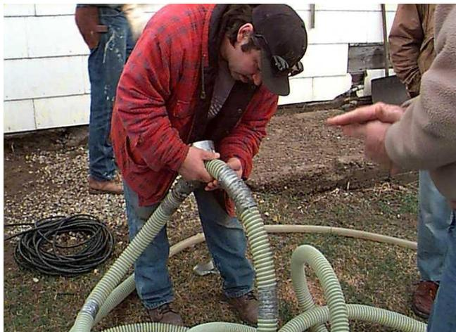
Sealing the hose leaks with duct tape is a good temporary solution. Butyl tape also works well. Clean the surface, apply the butyl tape and heat it with a torch to soften and seal. Tape over the butyl tape with duct tape to protect the seal and give it strength. A hose with many patches should be replaced.
