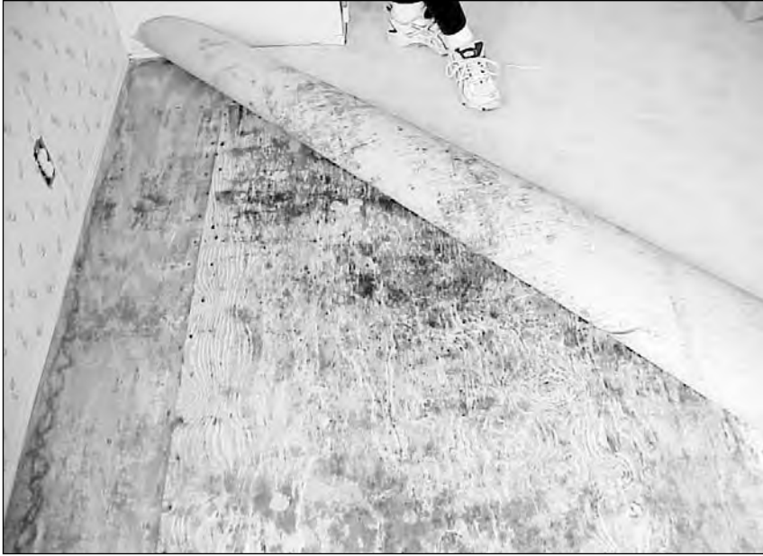
Vinyl flooring in manufactured homes can cause moisture damage, since the low moisture permeability of vinyl can lead to condensation.
