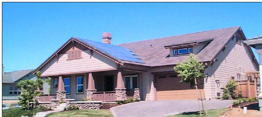
In addition to its improved design and NightBreeze cooling system, Centex Homes' "21st Century Performance Home" sports 3.6 kW of PV modules, making the house nearly a zero net user of electricity.
