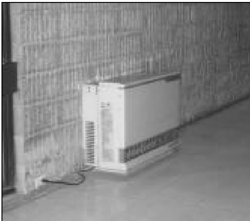
The Rinnai direct vent room heaters were chosen for their capacity modulation capability, which reduces oversizing-related cycling compared to constant-capacity heaters.
