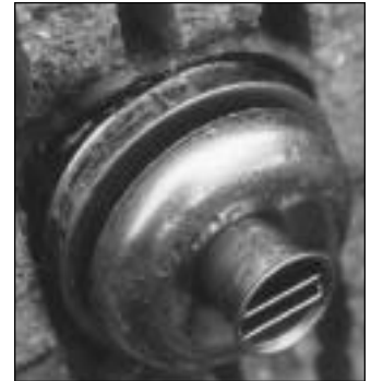
Vents must be located at least 9 inches below any window frame.
