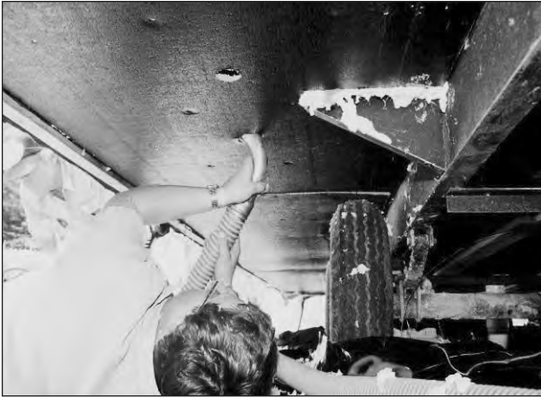
(left) To fill the outer area of the mobile home floor, a muffer pipe is attached to the flexible hose. The natural curve of the pipe makes it easy to rotate the pipe in the cavity to get maximum fill. (right) Batt stuffing is one way to reinsulate the walls of mobile homes. Remove the bottom two rows of screws, and you can stuff the insulation into the cavity using a strong, flexible plastic stuffer.
