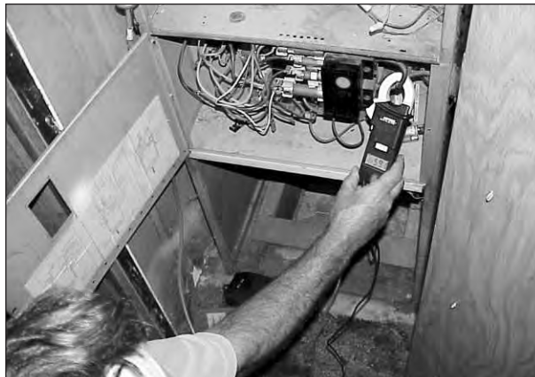
(left) Missing or badly damaged boots can be replaced to help air seal and increase the efficiency of the heating delivery system. (right) It is important to test the parts of an electric furnace. Many times, wires have been disconnected or improperly connected. This can pose a serious safety hazard.
