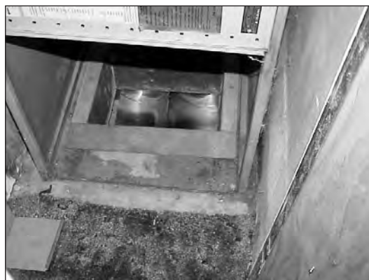
The plenum is a major area of air leakage. Too often when the mobile home is transported, movement causes the furnace plenum and the main duct run to separate, causing heat from the furnace to flow directly into the belly board instead of the ductwork.
