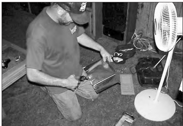
(left) Missing or badly damaged boots can be replaced to help air seal and increase the efficiency of the heating delivery system. (right) It is important to test the parts of an electric furnace. Many times, wires have been disconnected or improperly connected. This can pose a serious safety hazard.
