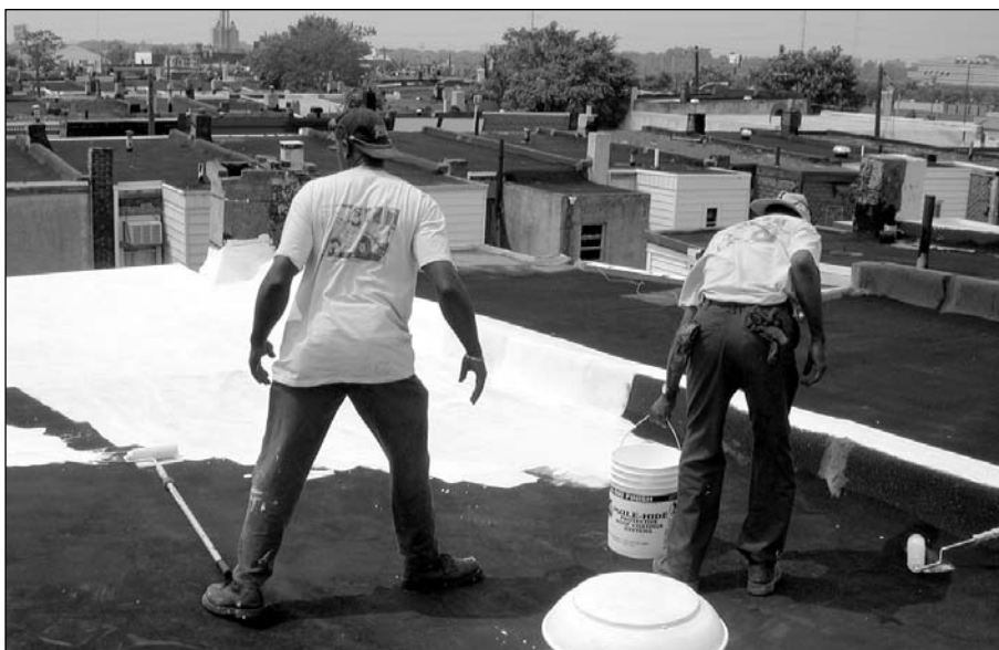
The coating that is being applied protects the roof from ultraviolet radiation, which breaks down the asphalt roofing material.
