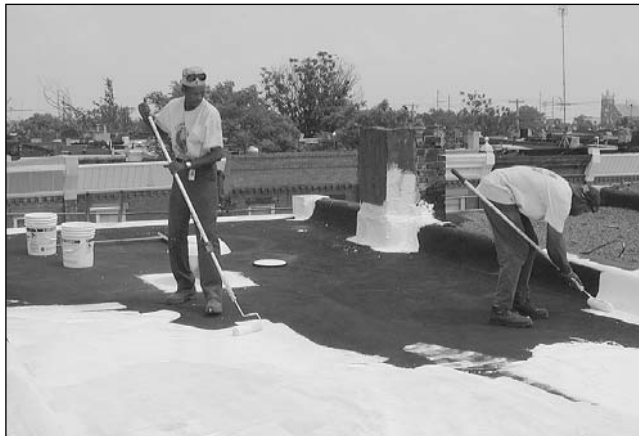
An ECA crew applies white acrylic elastomeric roof coating on a Philadelphia building using simple tools—rollers.
