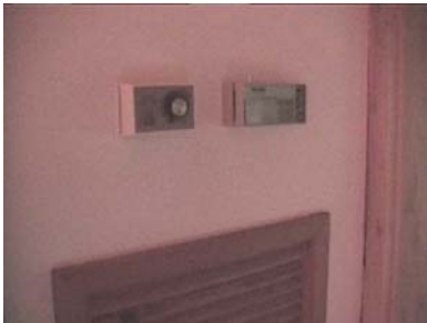
Thermostat and Humidistat on Bypass Wall
