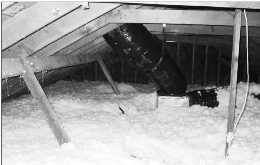
The new flex ducts in the attic are covered by additional blown-in insulation after the retrofit.
