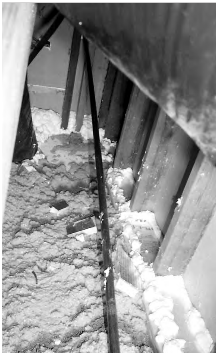
It's important to seal cavities connecting the house to the attic. Foam was used for sealing small holes and cracks at building component intersections.
