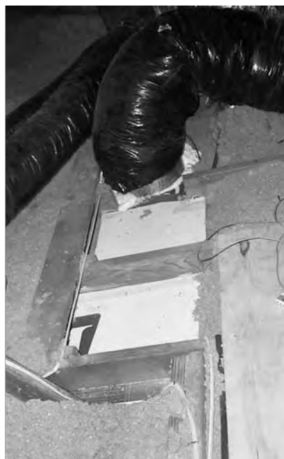
Duct board insulation was used to block off large open areas.
