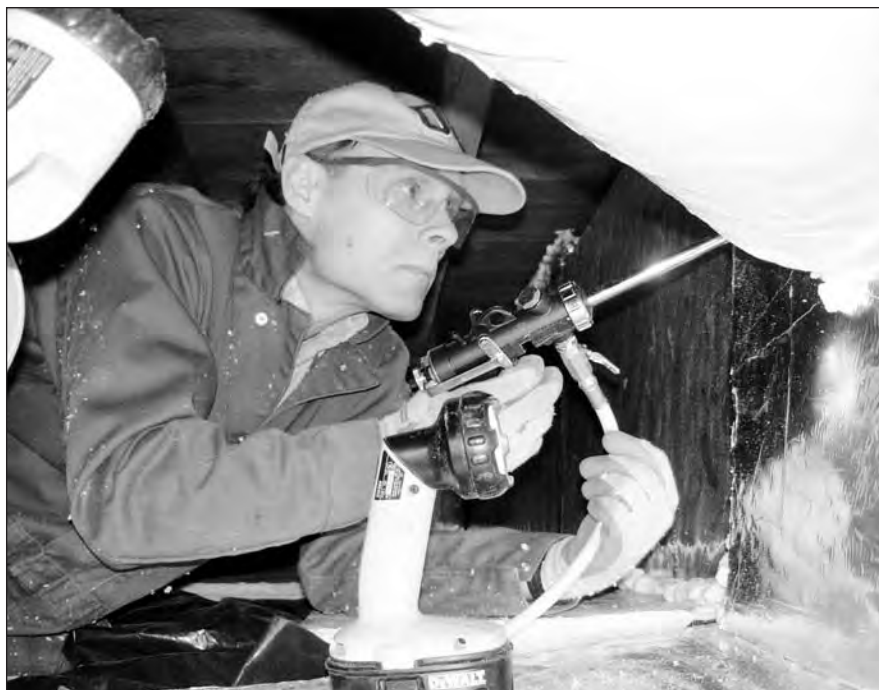
Building Science Corporation's Nathan Yost seals a crawlspace.
