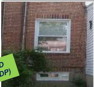
Energy Star windows installed
