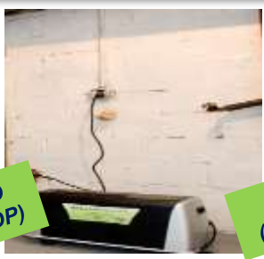
Mold remediated; dehumidifier installed
