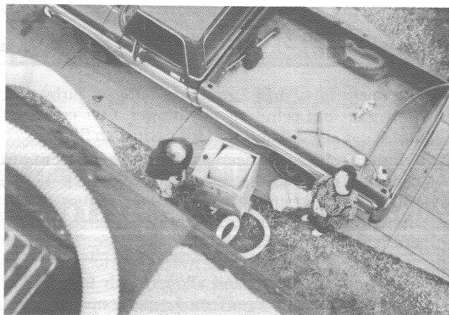
The homeowner looks on as Gary adjusts the settings on the blower for the hoser on the roof.
