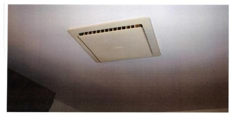
Existing fans tested at 16-20 cfm and disconnected in attic
