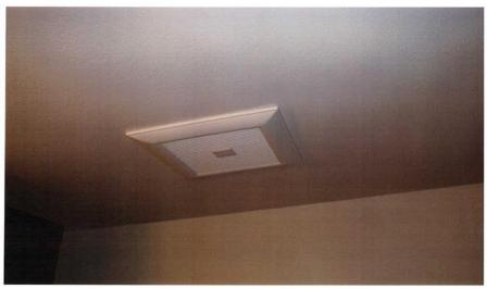
New fans installed tested at 80+CFM set on continuous run per ASHRAE Standards
