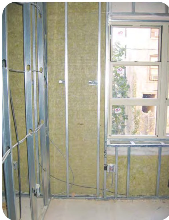
The building walls are insulated with R-4.3 Roxul 1-inch rigid (mineral wool) insulation and R-13 fiberglass batts within 3 1/2-inch interior steel framing. The rigid insulation, placed between the steel studs and the CMU block wall, minimizes thermal bridging through the steel.
