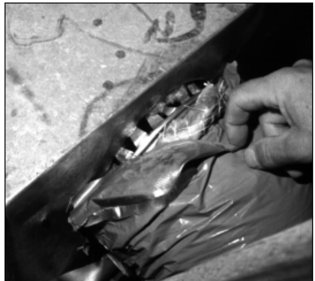
Supply Leak at Take-Off Connection
