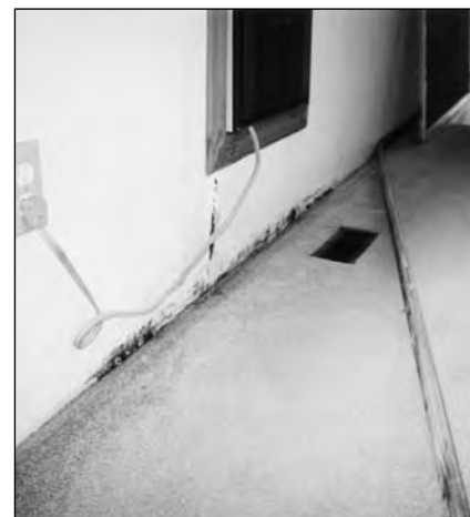
(left) The cracking drywall implies a moisture problem. (right) Removing some baseboard reveals the first signs of mold.
