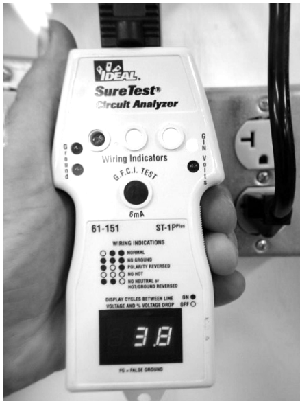
SureTest Circuit Analyzer showing a voltage drop of 3.8% (receptacle model 61-151 / ST-1P plus)
