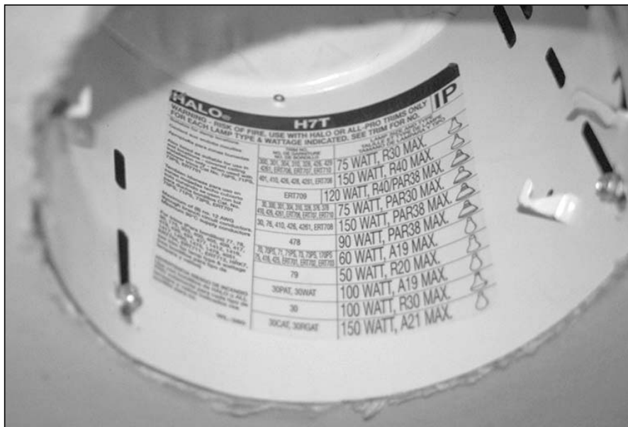
Manufacturers' trim and bulb recommendations are printed on the recessed-can housing.
