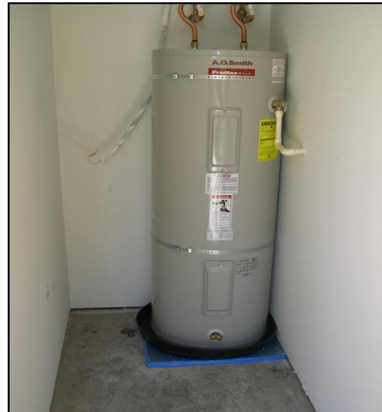
Hot water heater, drip pan, insulated under
