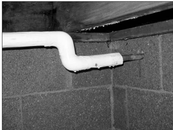
This is an example of a wet crawlspace—notice the water dripping off of the pipe insulation.
