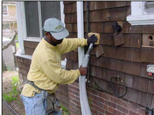
**The one-hole method using a tube long enough to reach to the furthest corner of the cavity is the best way to dense pack walls**
