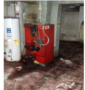
Broken hot water heater and furnace
