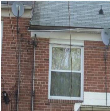
Defective gutters causing water leaks
