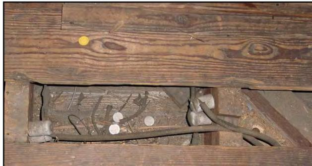
**Even if there is attic flooring, knob-and-tube wiring and attic bypasses must be found and treated before insulation is added**
