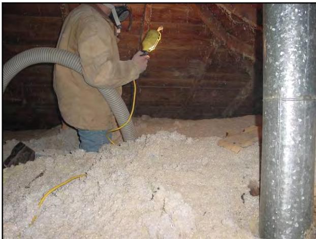
Do not blow loose-fill insulation tight against roof deck over top plates. Cellulose should not be specified where it may come in contact with exposed metal roofing.
