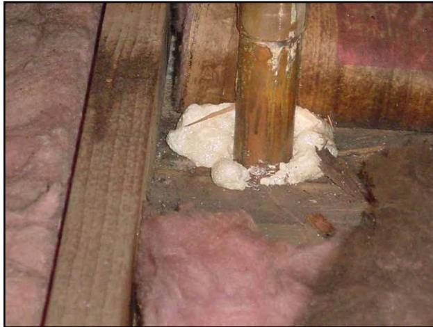
**Plumbing stack sealed with foam**
